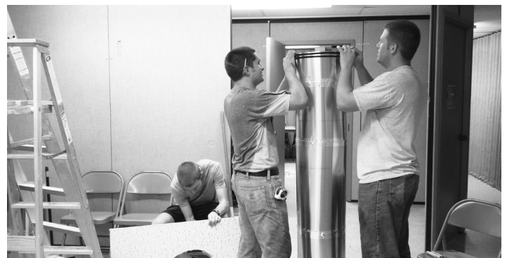
Daniel Graber, Mark Bowman, and Aaron Lehman install one of three solar panels.
