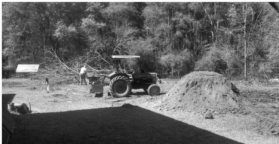
Ed Swartzendruber clears an old well shed and trees to prepare space for a new pole barn. The first of four loads of dirt which Ed spread and leveled for the building pad awaits his attention.
